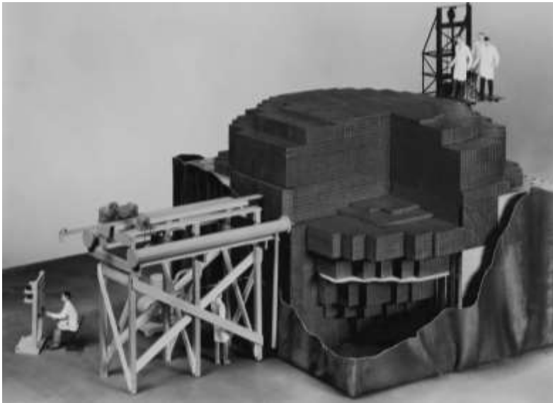
Figure 1-4. Cutaway view of ChicagoPile-1 showing the graphite blocks
