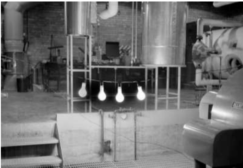
Figure 1-10. EBR-I produced the first electricity from nuclear, supplying power to the reactor control system as well as the building and a machine shop
